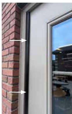
CONTINUOUS HINGE - CLOSED
