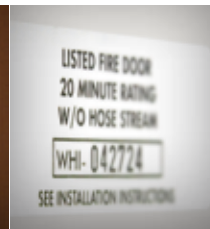
Listed Fire Door 20 Minute Rating (with specialty core)
