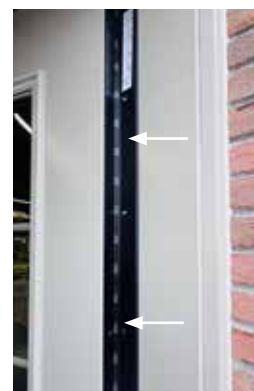
CONTINUOUS HINGE - OPEN
