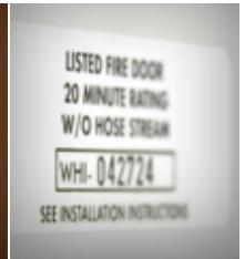
Listed Fire Door 20 Minute Rating (with specialty core)
