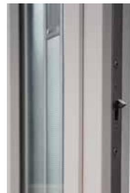
Multi-Point Locking System on Venting Sidelite
