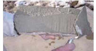
"Back-butter" the back of the stone with mortar before attaching to the scratch coat.
