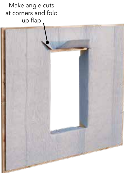
1. Cut modified "H" in housewrap
