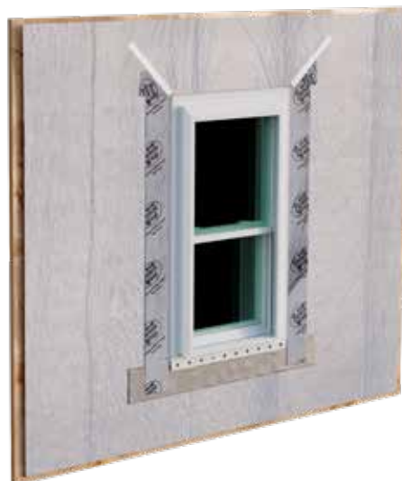
5. Tape cuts over head flashing
