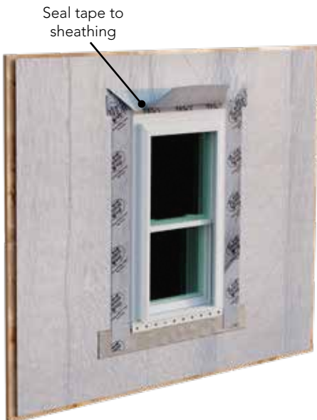
4. Apply head flashing
